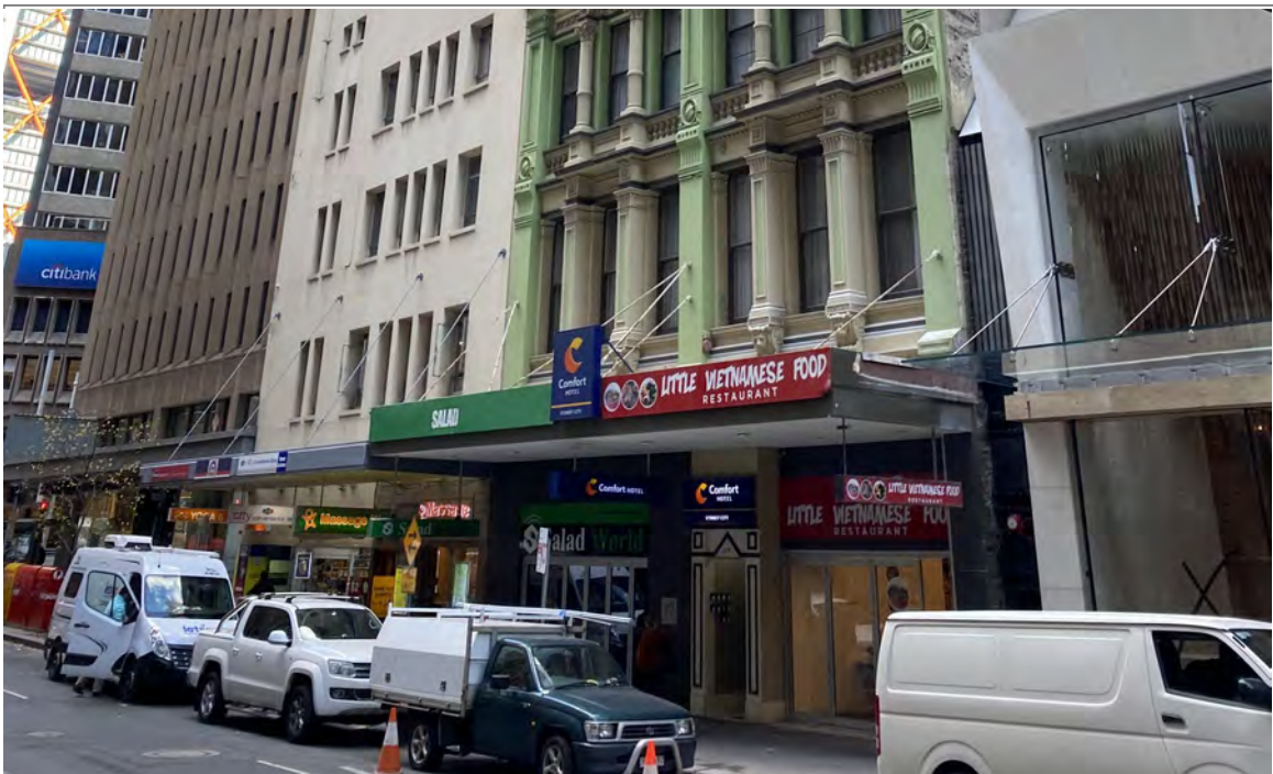
Photo 10: Hunter Street look towards the south to 15 Hunter Street
